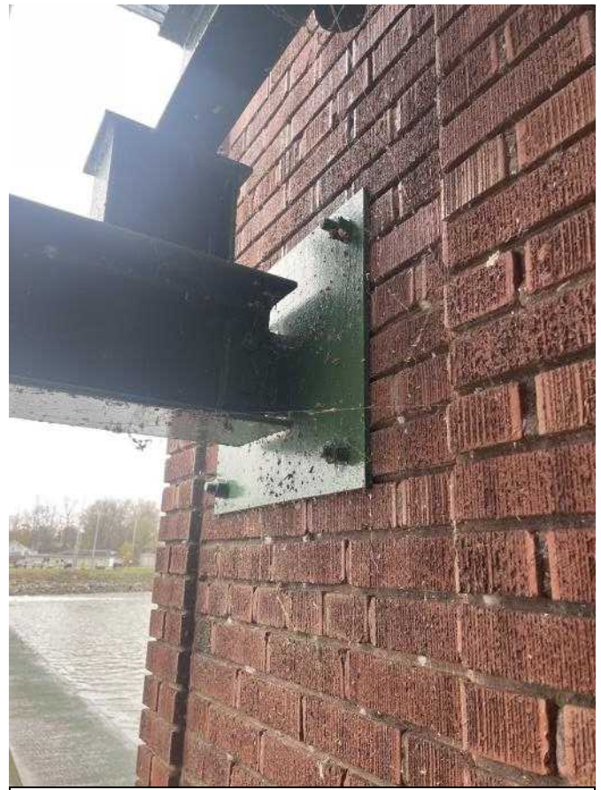
Photo 0060811042470 - Slide gate platform with anchor to
