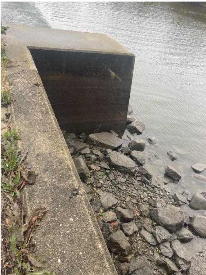
Photo 0060811042451 - West spillway abutment and riprap
