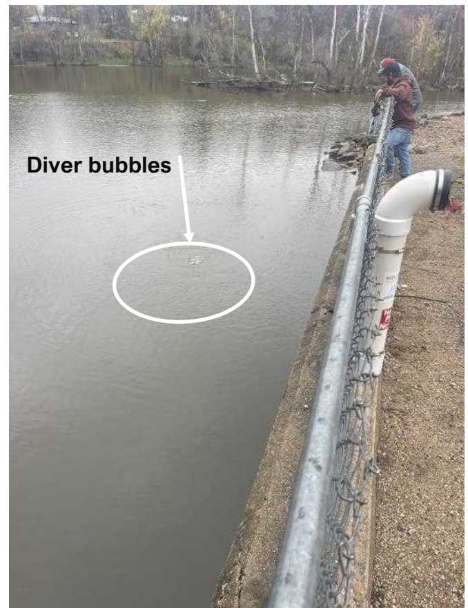
Photo 0060811042444 - East retaining wall inspection
