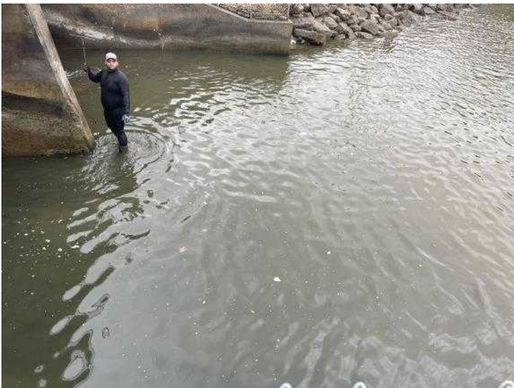
Photo 0060811042416 - Diver inspection of auxiliary gate abutments
