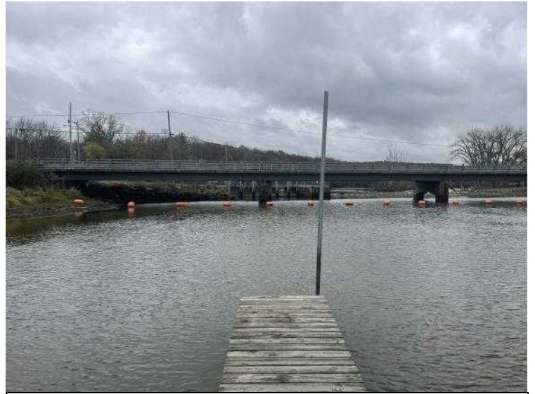
Photo 0060811042403 - Auxiliary slide gate area (looking south)
