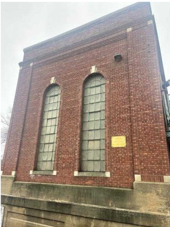
Photo 0060811042455 - Power house east wall
