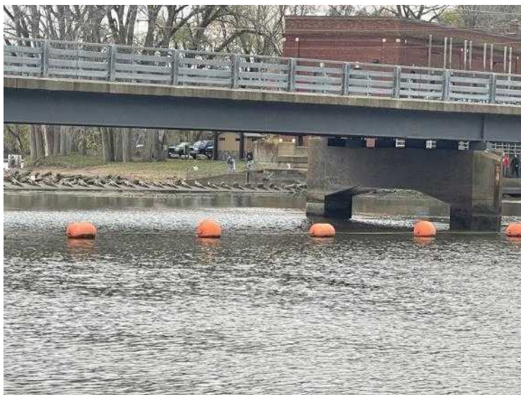
Photo 0060811042404 - Spillway (looking south)
