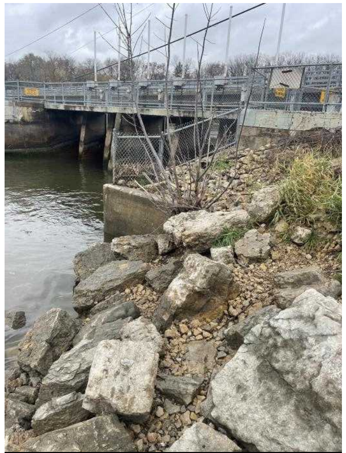
Photo 0060811042419 - Auxiliary gate and adjacent riprap
