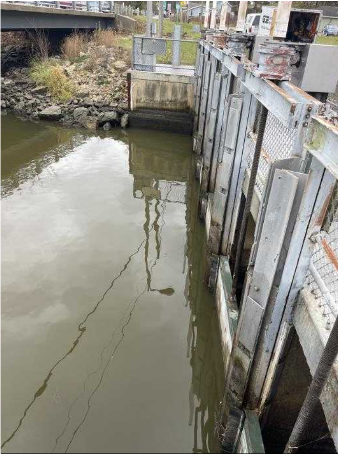
Photo 00608110424010 - Auxiliary side gate up river
