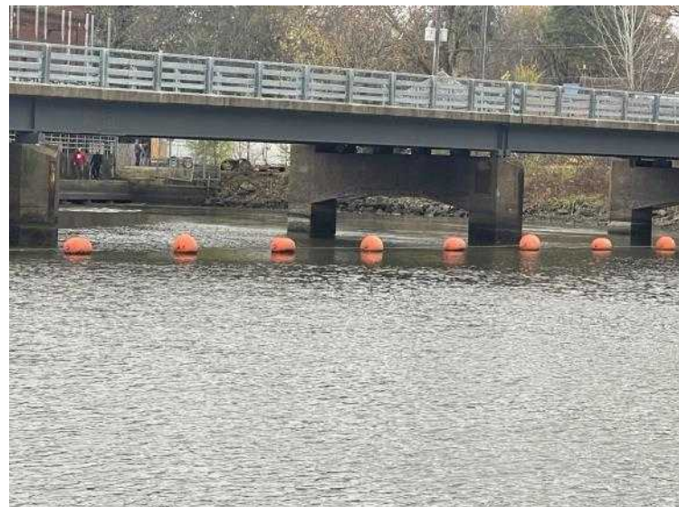
Photo 0060811042405 - Power house building slide gates
