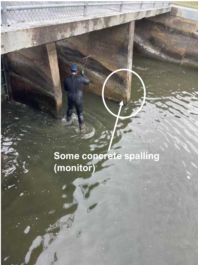
Photo 0060811042414 - Diver inspection of auxiliary gate
