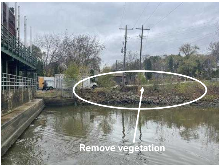
Photo 0060811042438 - West bank up stream of power house
