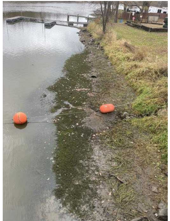
Photo 0060811042424 - Up river from auxiliary slide gates
