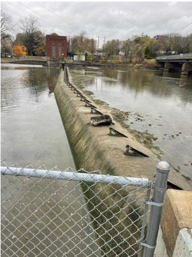
Photo 0060811042408 - Center spillway looking east
