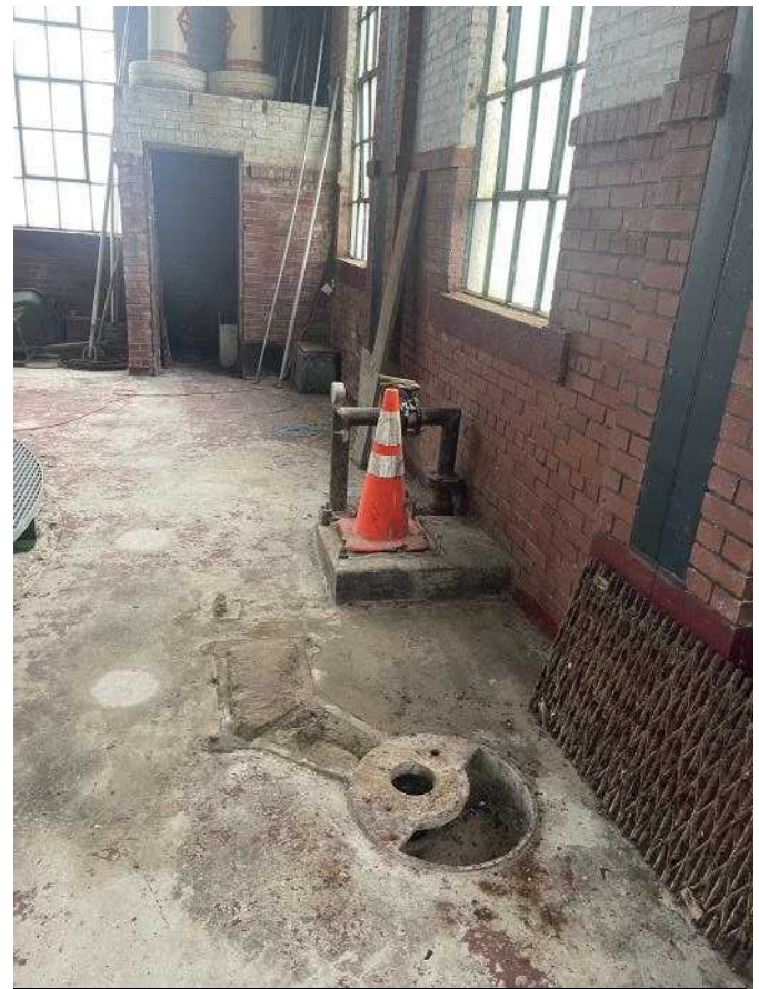
Photo 0060811042460 - Power house south wall
