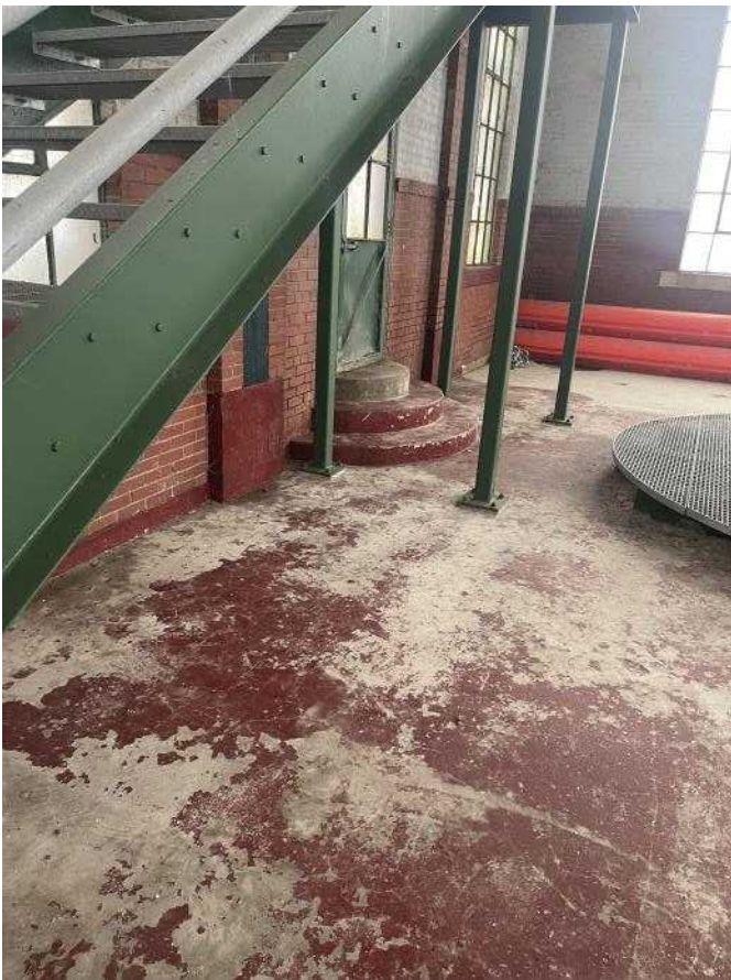
Photo 0060811042459 - Power house north wall (looking east)
