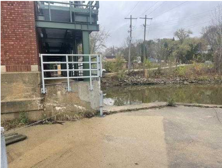
Photo 0060811042457 - Power house slide gate (bay number 6)
