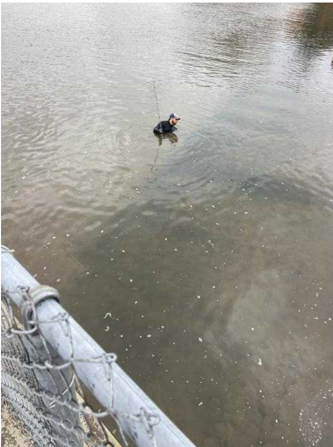
Photo 0060811042412 - Diver inspection of spillway apron
