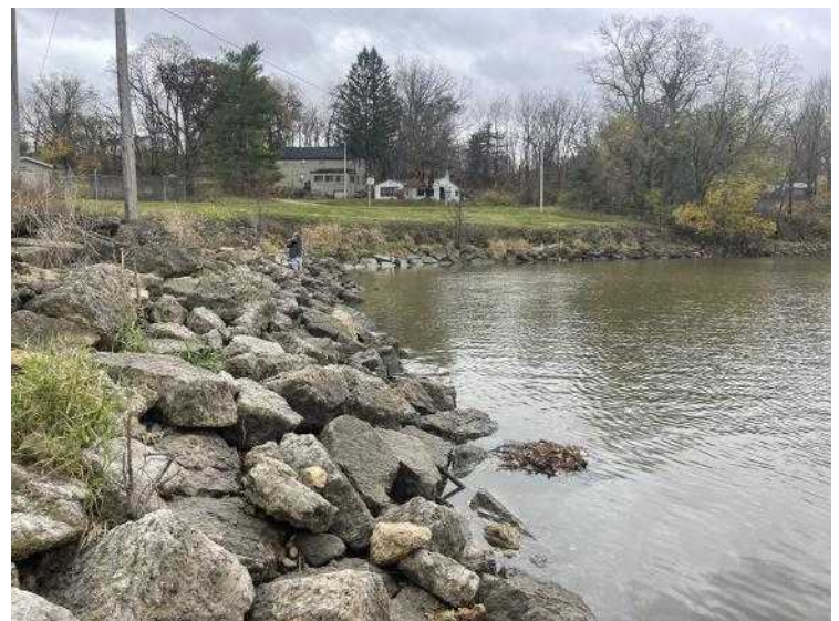
Photo 0060811042421 - Auxiliary gate riprap looking east. No signs of seepage. Above ground scope stable with 2-3 foot wide riprap
