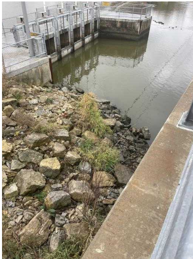
Photo 0060811042422 - Riprap of auxiliary gate between
