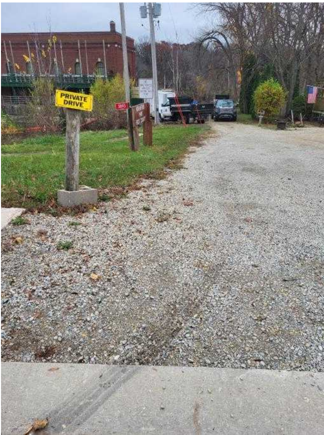
Photo 0060811042472- Access road way at power house
