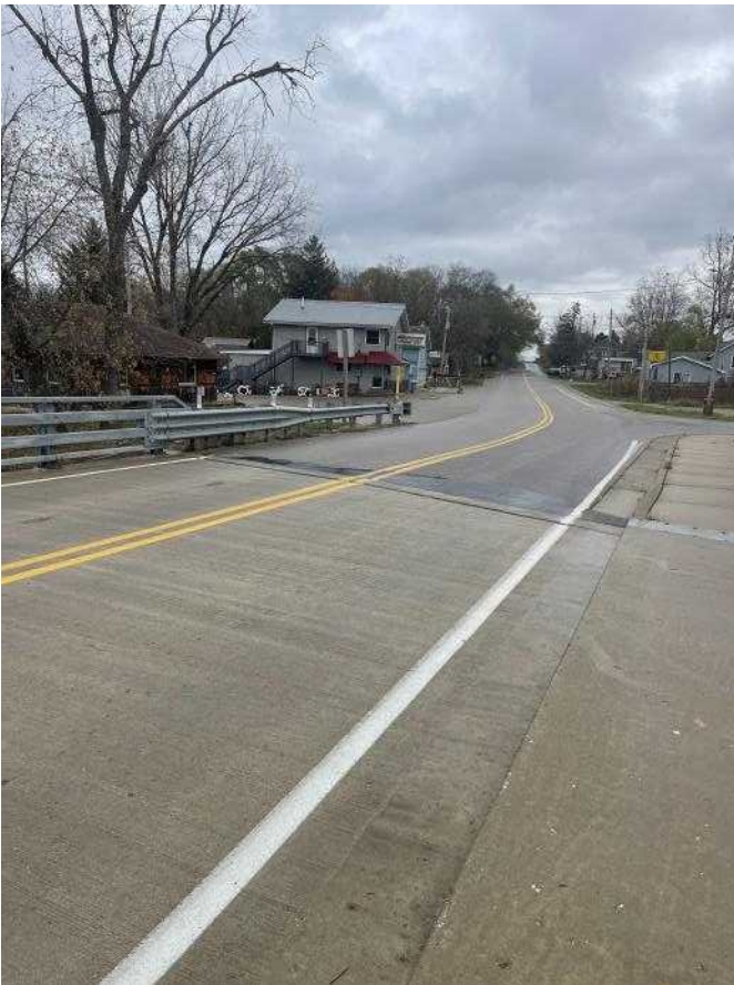
Photo 0060811042423 - County Road M looking east at
