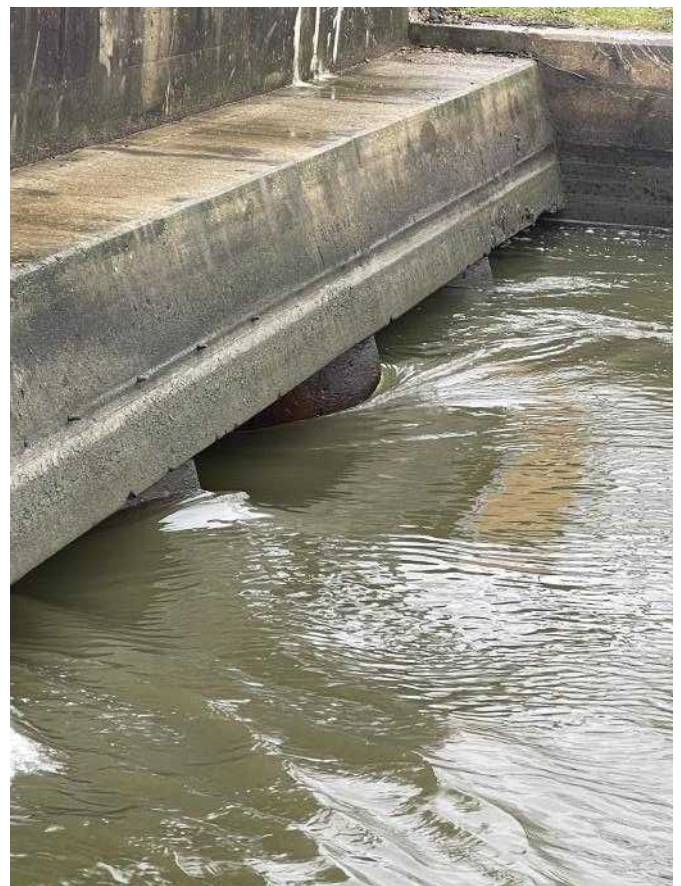
Photo 0060811042437 - Power house up stream wall
