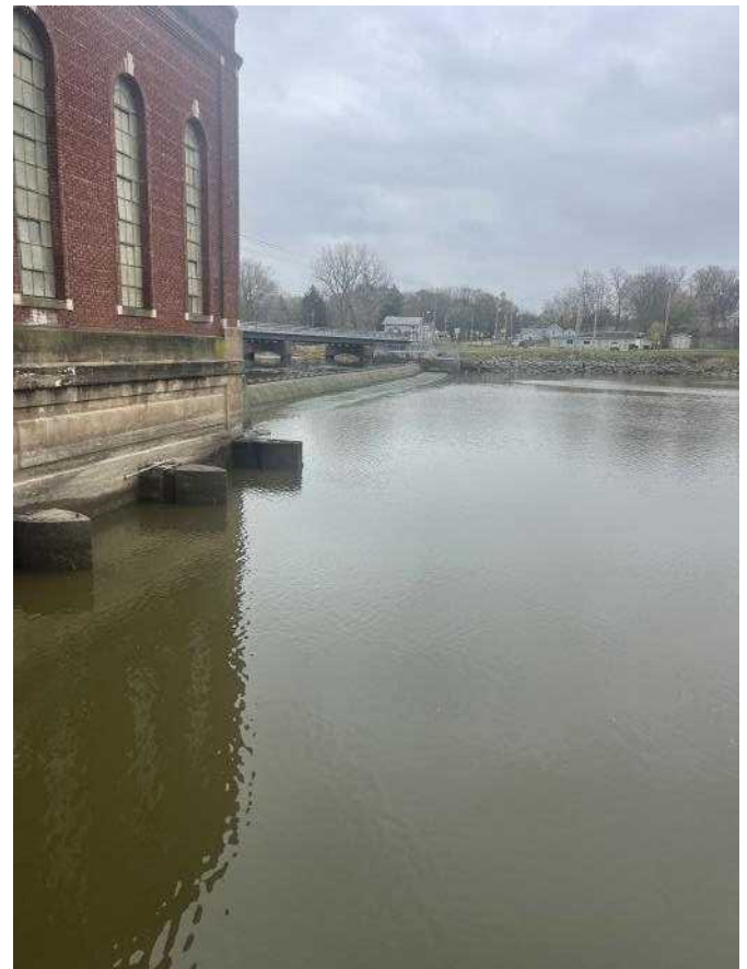
Photo 0060811042448 - Inspection of east gates bays 1 and 2
