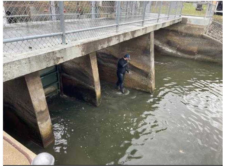
Photo 0060811042415 - Diver inspection of auxiliary gate abutments
