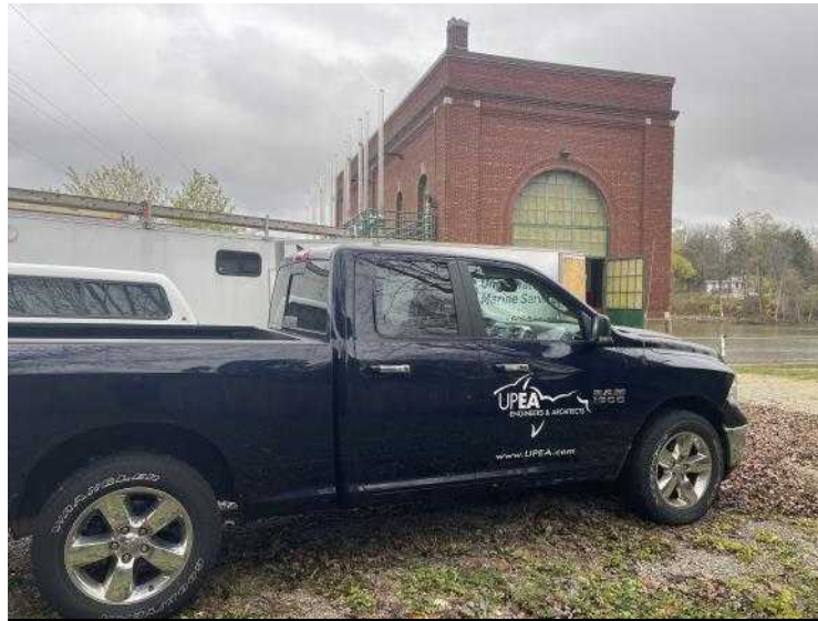
Photo 0060811042442 - Power house (looking east)
