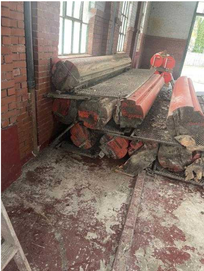
Photo 0060811042461 - Power house south wall
