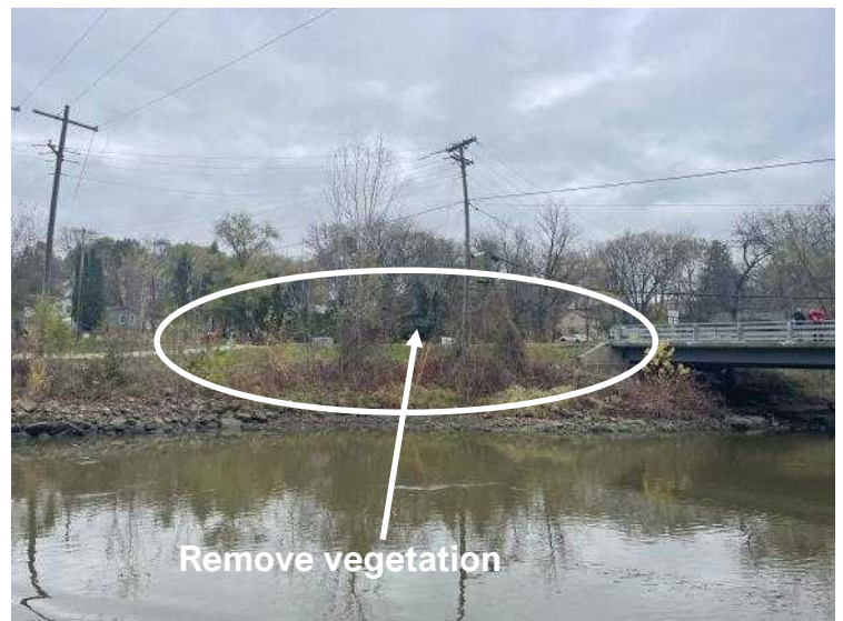
Photo 0060811042439 - West bank upstream of power house
