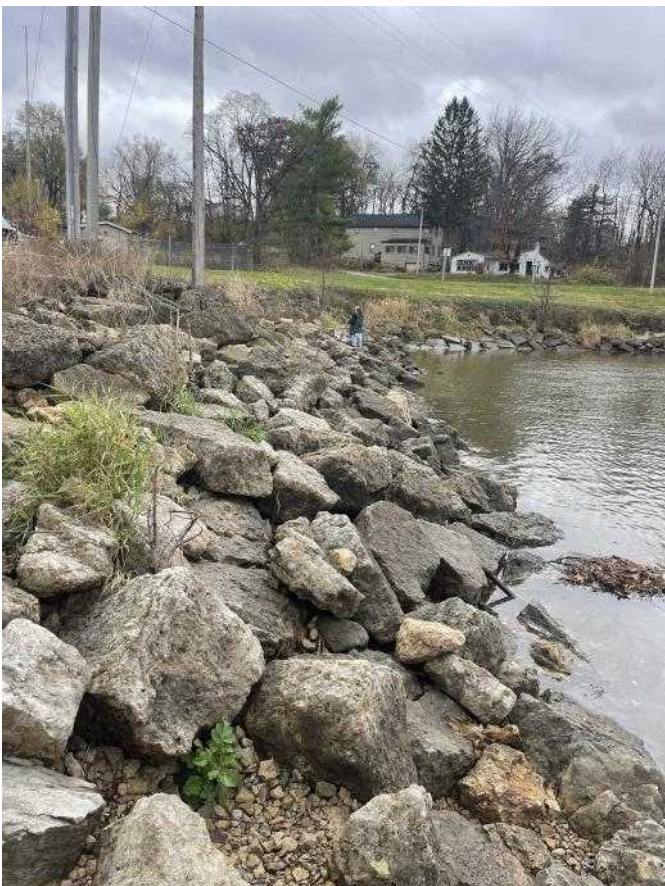
Photo 0060811042420 - Auxiliary gate riprap (looking east)
