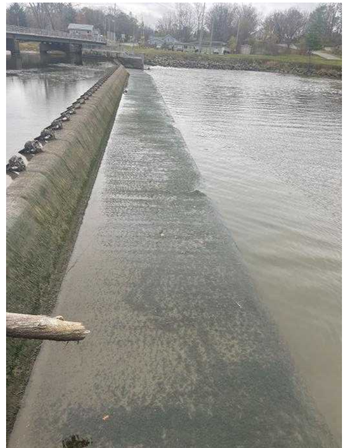
Photo 0060811042452 - Main spillway and apron
