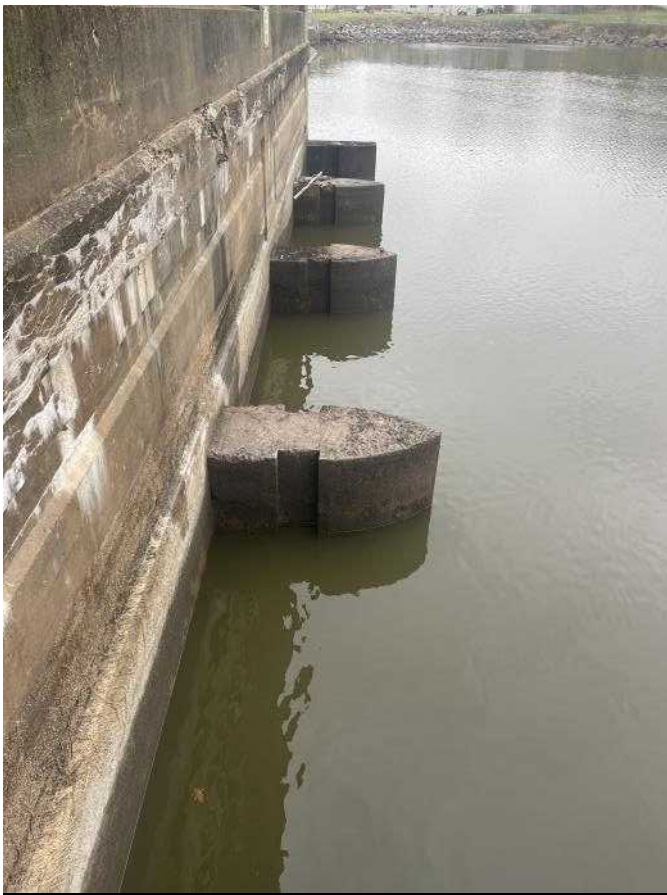
Photo 0060811042445 - Power house inspection
