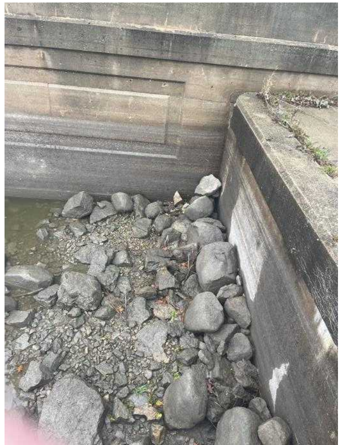
Photo 0060811042450 - Down stream riprap east of power
