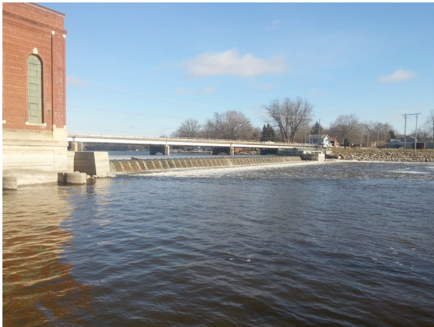
Photo 0060812051303 – Downstream face of dam
