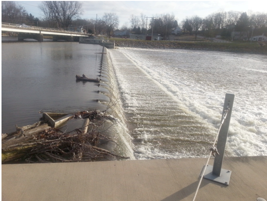
Photo 0060812051301 – View along crest of dam
