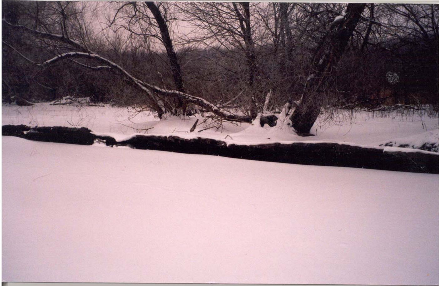
Winter erosion on Carcajou Point. Ice under tree root systems due to low water levels. Undercutting of tree root systems as ice sheet shifts.
