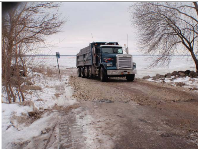
At the tracking pad, looking south.
