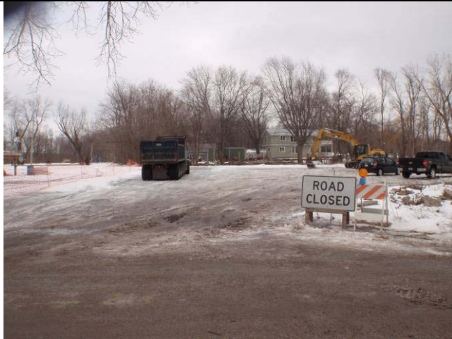
At the entrance of the staging area, looking NE.
