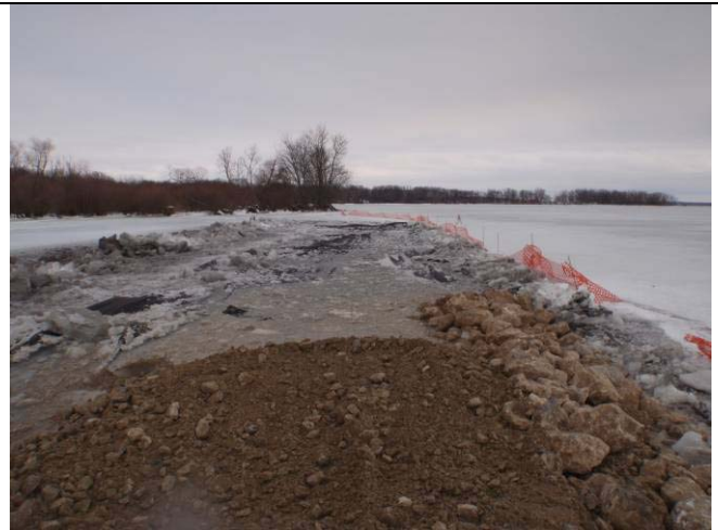
At the southern end of the completed berm looking NW.
