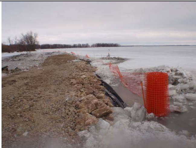
At the north end of the berm looking NW.
