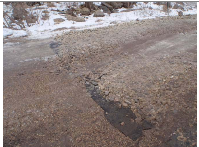
Close up of the geotextile underneath the tracking pad.
