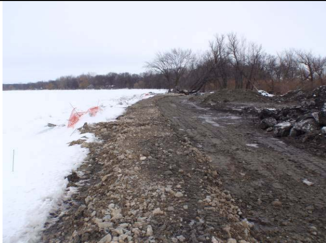
At the center the berm looking north.
