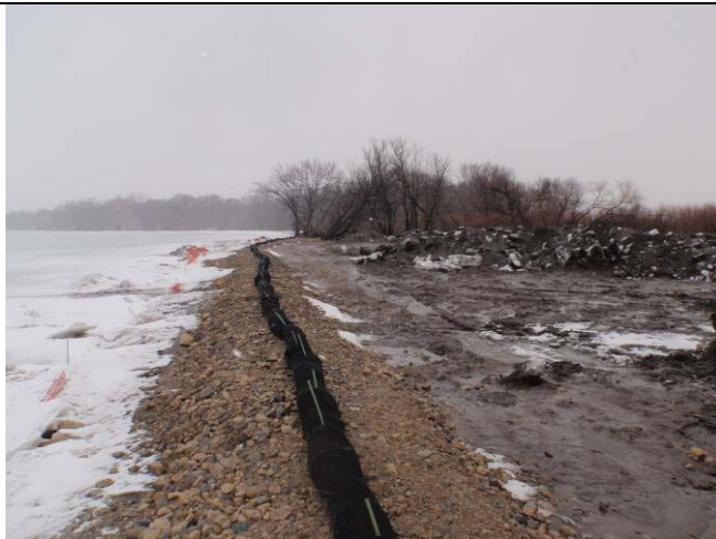
At the center the berm looking north.
