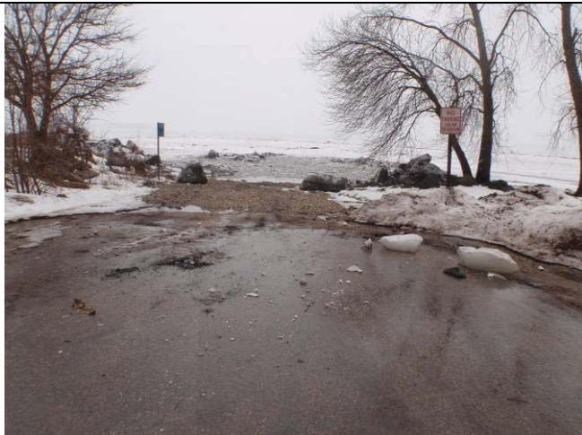
At the tracking pad, looking south.
