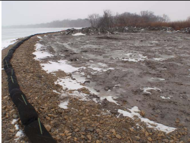
At the south end of the berm looking north onto the dredge placement area.
