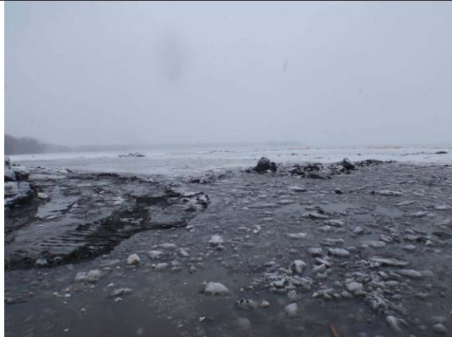
At the boat launch, looking east onto the eastern side of the dredge area.
