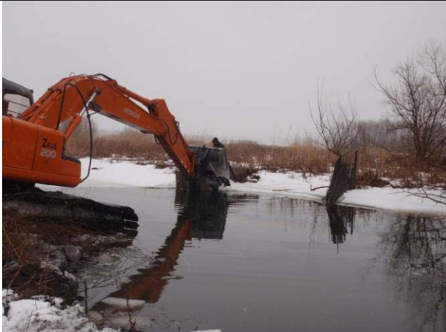
At the carp gate looking north onto the construction.
