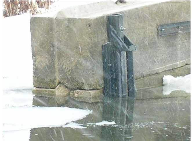
At the carp gate looking east onto the installed east anchorage.
