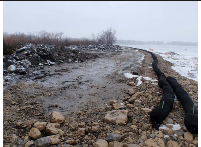
At the north end of the berm looking south onto the dredge placement area. The two portions of the silt sock has been temporarily moved for vehicle access.
