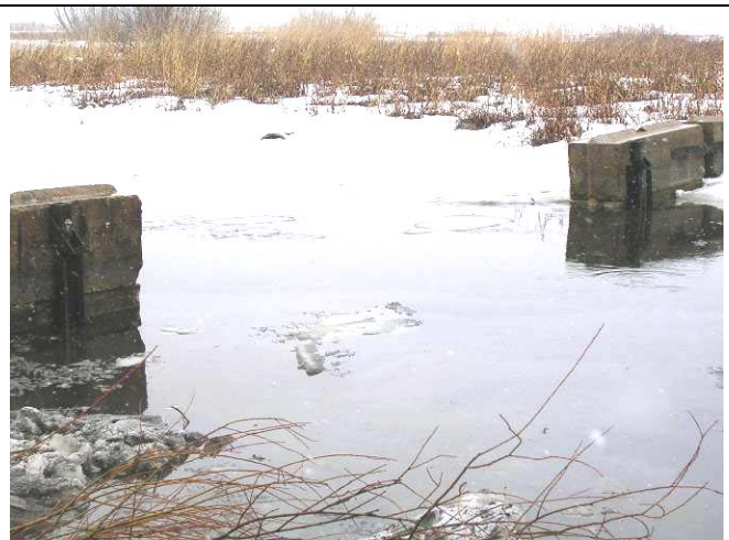
At the carp gate looking north onto the installed anchorage.
