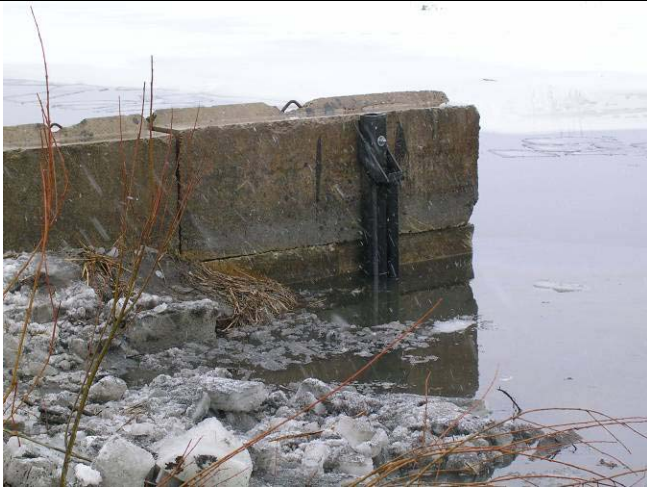
At the carp gate looking east onto the installed west anchorage.
