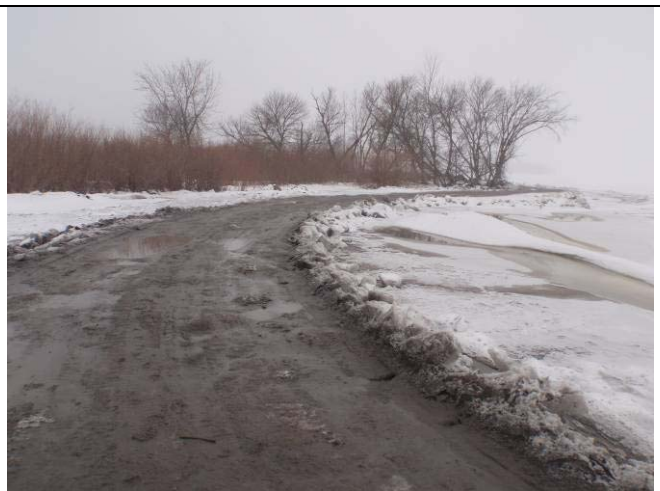
Looking south toward the north end of the berm.
