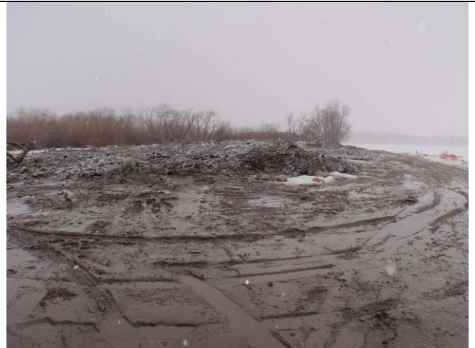
At the north end of the berm looking south onto the dredge placement area.
