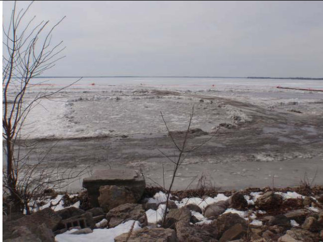
At the staging area, looking south onto the center of the dredge area.
