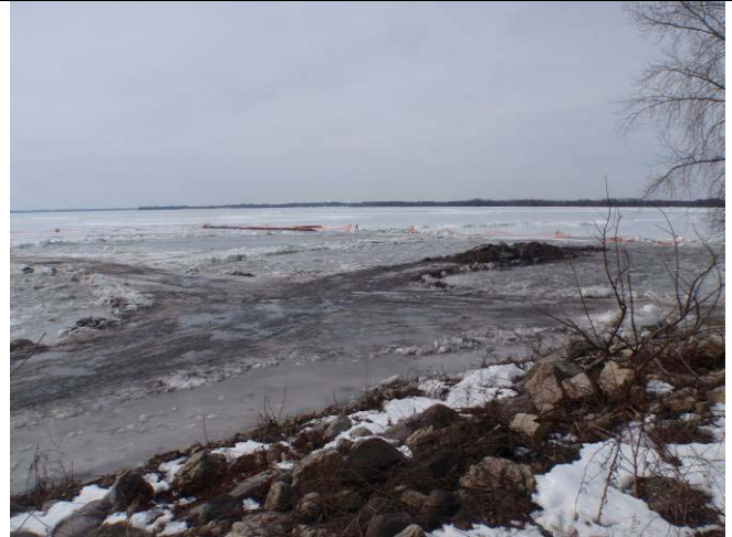
At the staging area, looking west onto the western side of the dredge area.
