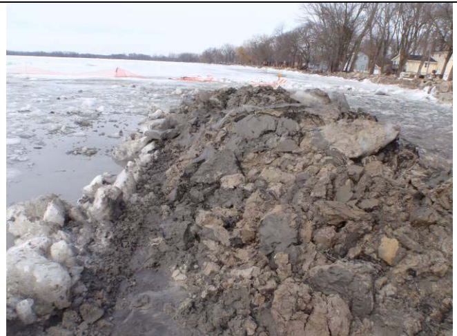
Close-up of the dredge spoils pile.
