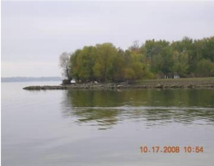
Photograph of rock armor extending west towards Carcajou Point. Rock armor appears to be maintaining position and effectiveness.
